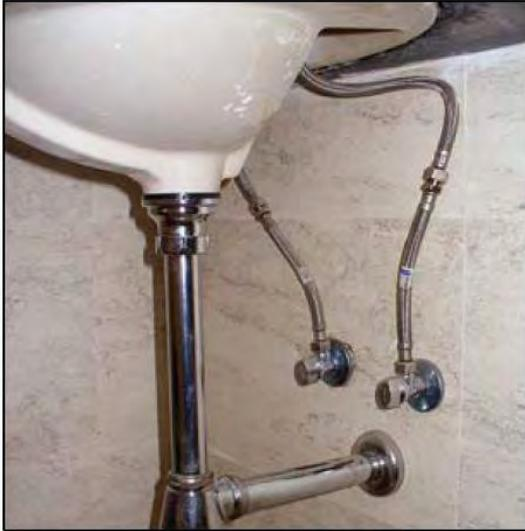
**Fig 3.** Conectores flexibles
