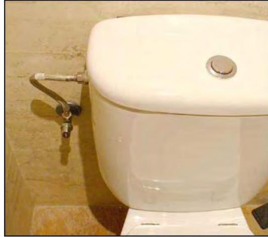
**Fig 4.** Conectores flexibles
